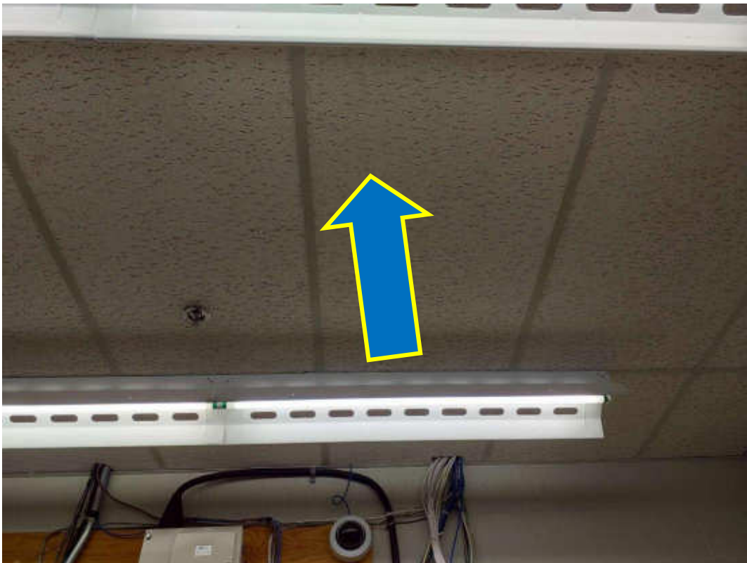
V9500 (Presumed Asbestos), 24x48 long widthwise fissure, Ceiling, Ceiling Tiles (lay-in), Mechanical P/House (Location #: 295) Server room
