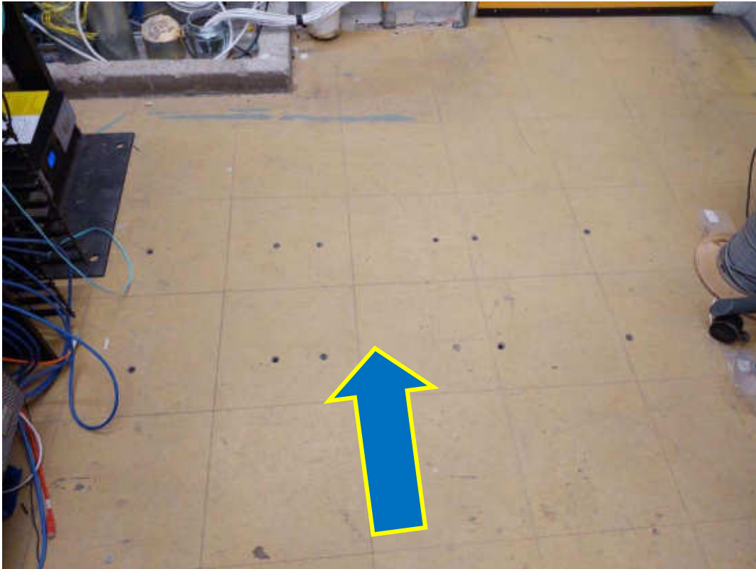
V9500 (Presumed Asbestos), 12x12 yellow, Floor, Vinyl Floor Tile, Mechanical P/House (Location #: 295) Server room
