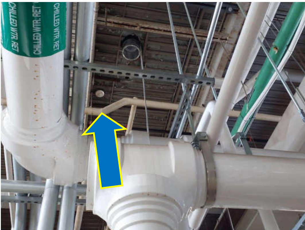
S0008 (Confirmed Asbestos), Piping, Parging Cement, Boiler Room (Location #: 1)
