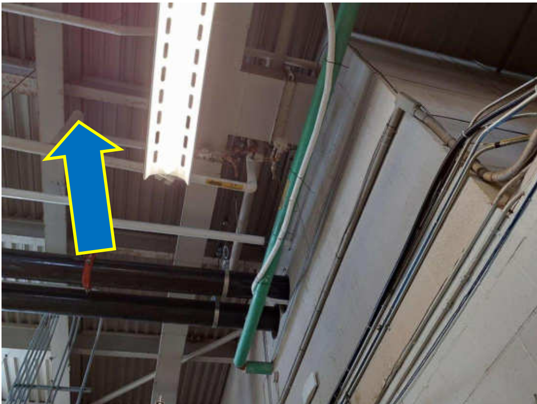
S0007 (Confirmed Asbestos), Piping, Parging Cement, Boiler Room (Location #: 1)
