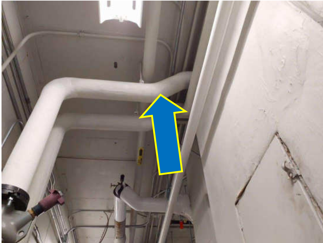
S0075 (Confirmed Asbestos), Piping, Parging Cement, Mechanical P/House (Location #: 295)
