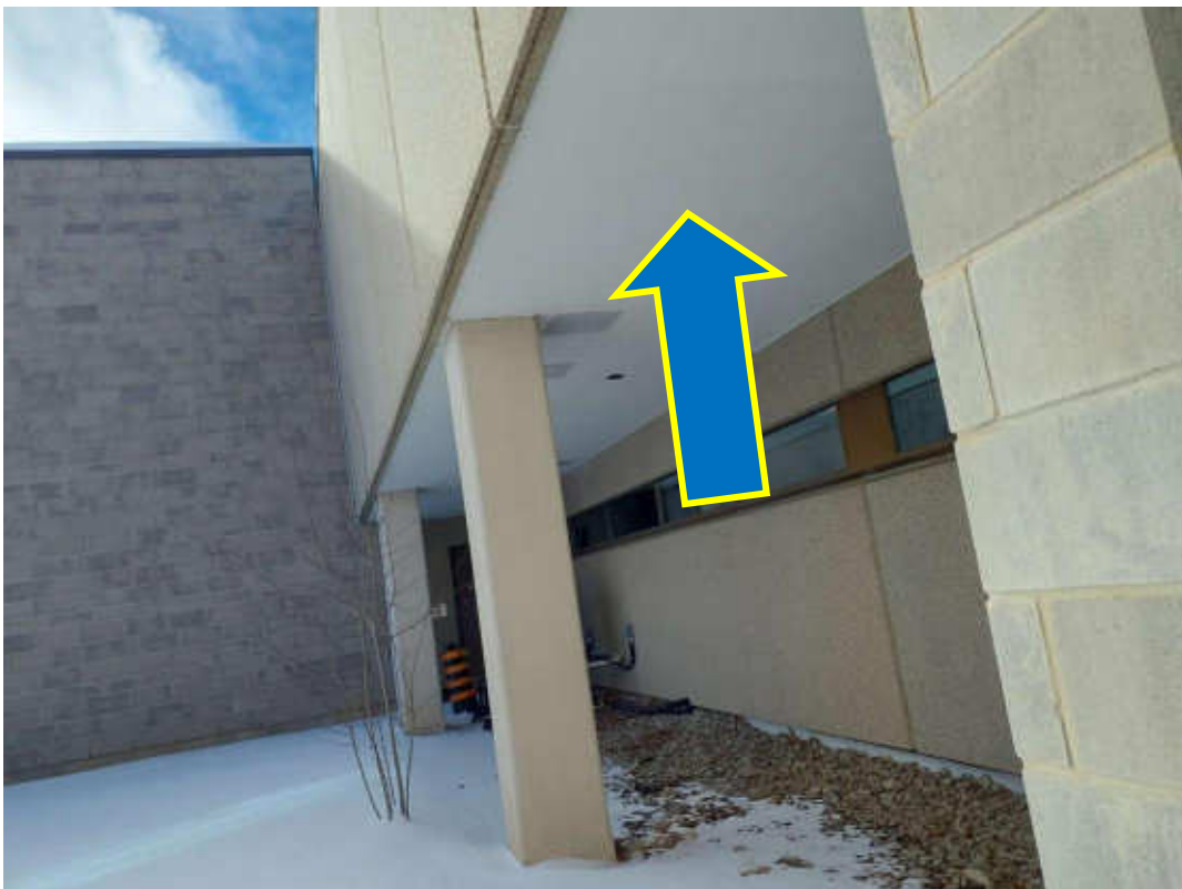
S0073 (Confirmed Asbestos), Ceiling, Texture Coat, Exterior Soffit (Location #: 296)
