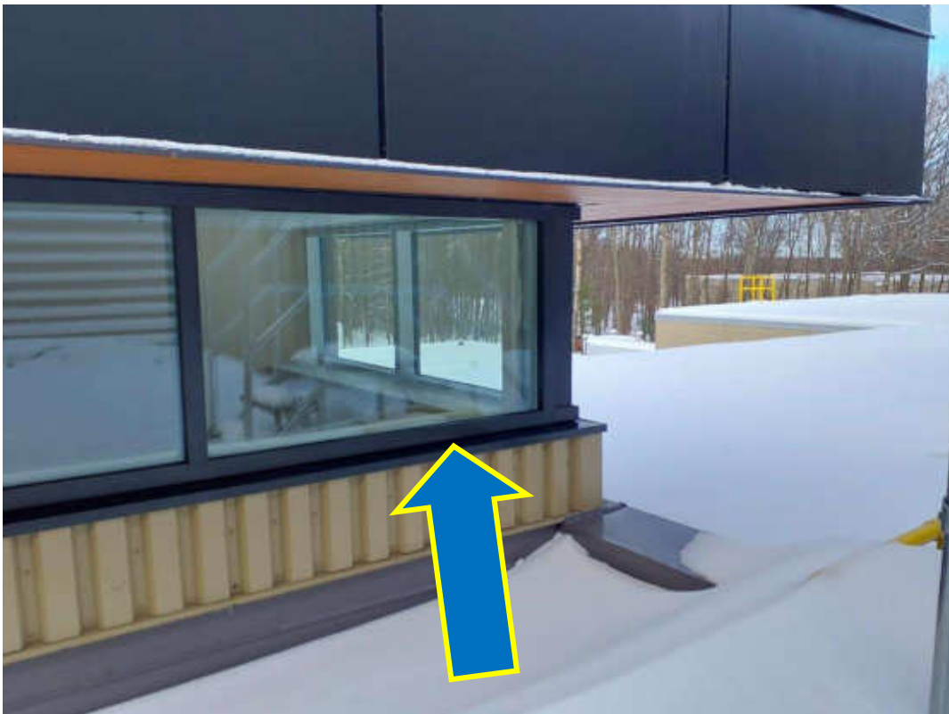
V9500 (Presumed Asbestos), Black on window base plate, Wall, Caulking, Roof Section D2 (Location #: 315)
