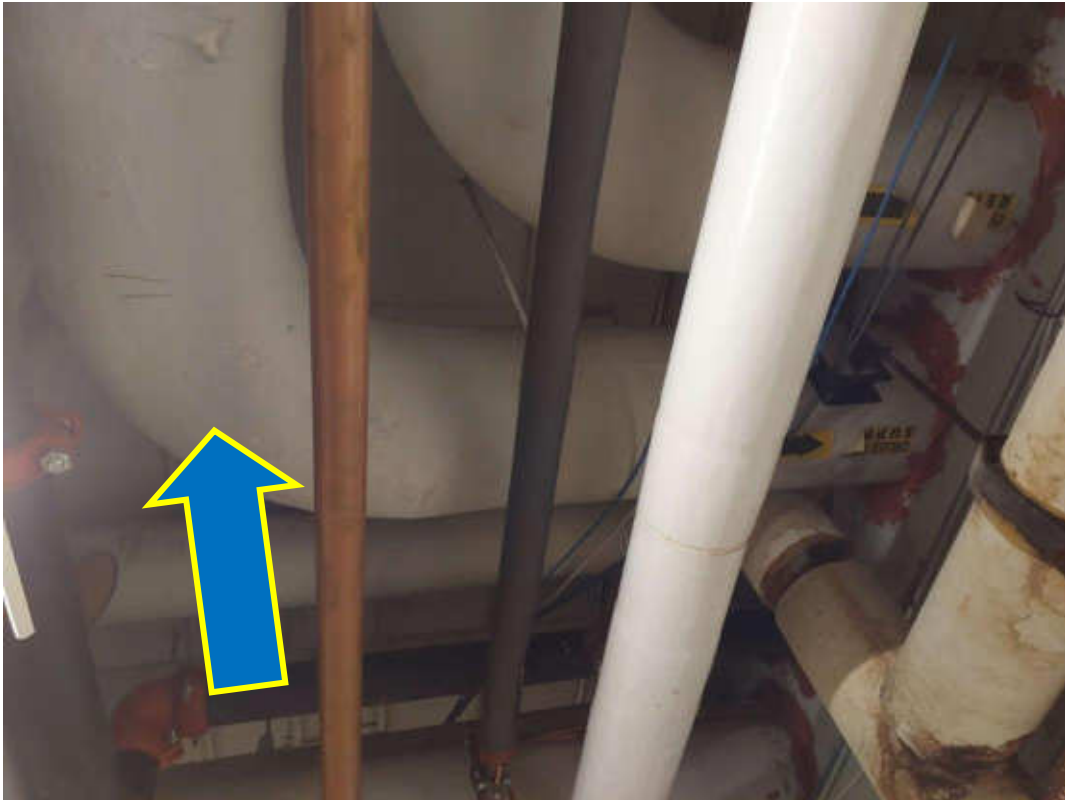
V0001 (Confirmed Asbestos), Piping, Domestic Cold Water, Parging Cement, Corridor (Location #: 10)
