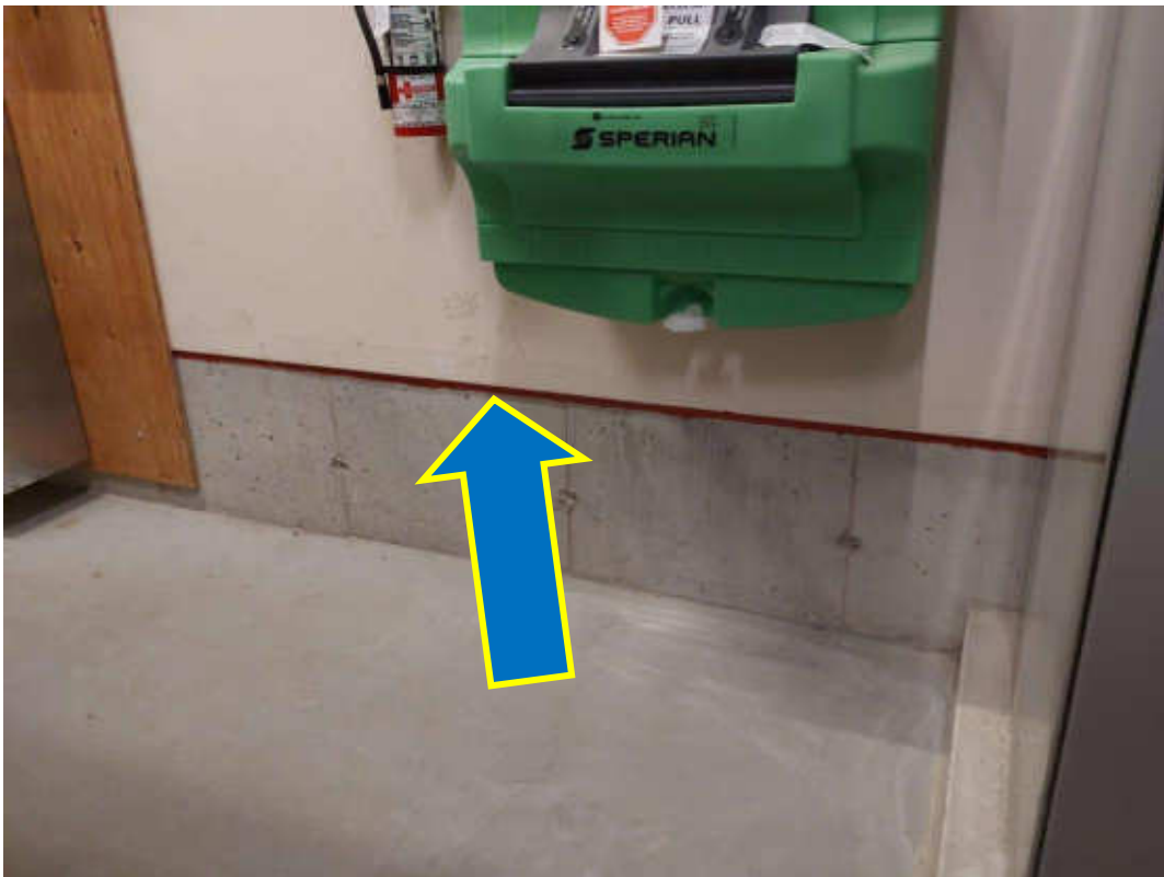
V9500 (Presumed Asbestos), Red at drywall wall edges and pipe penetrations, Other, Firestopping (mastic), Mechanical P/House (Location #: 295)
