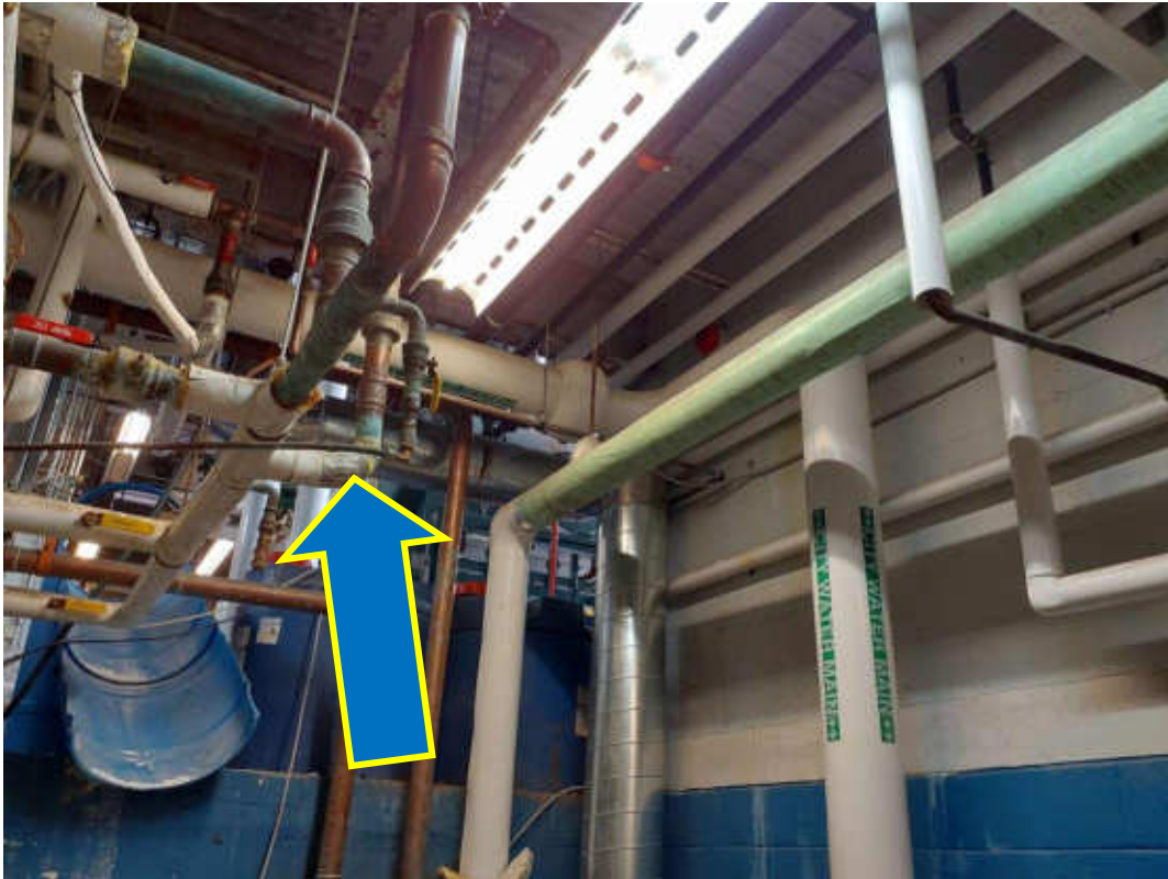
V0002 (Confirmed Asbestos), Piping, Parging Cement, Lower Boiler Pits (Location #: 8)
