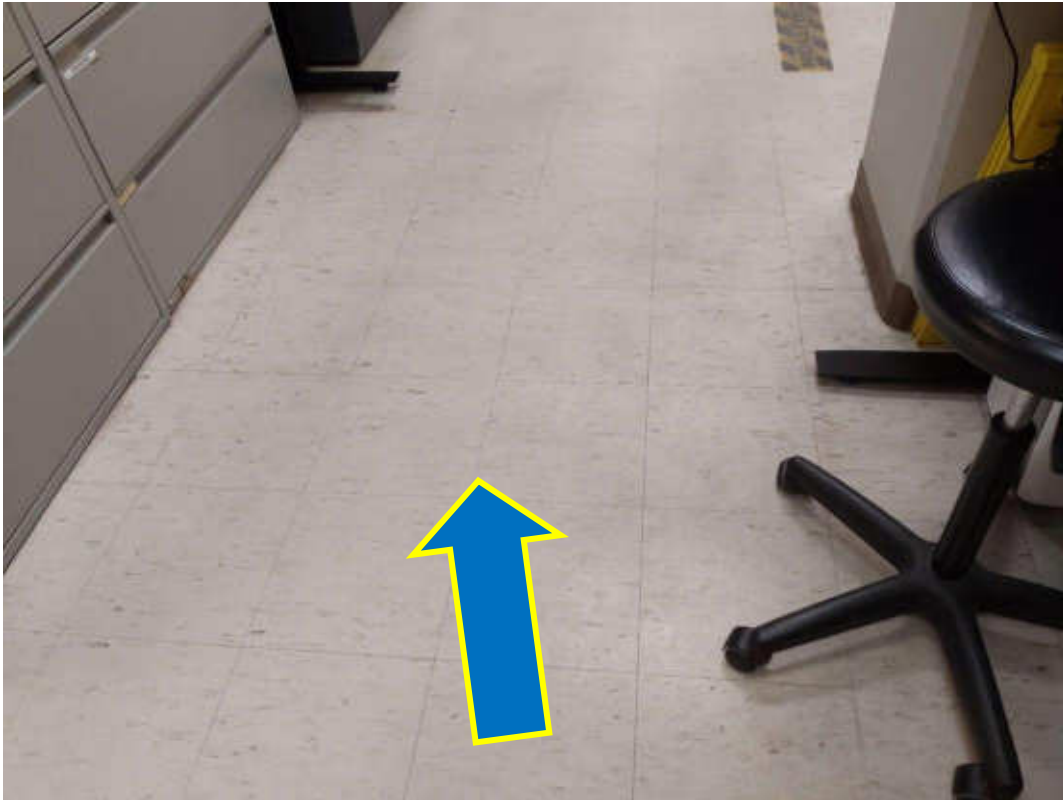
S1101A (Confirmed Asbestos), 12"x12" grey with grey streaks, Floor, Vinyl Floor Tile and Mastic, Pharmacy (Location #: 38)
