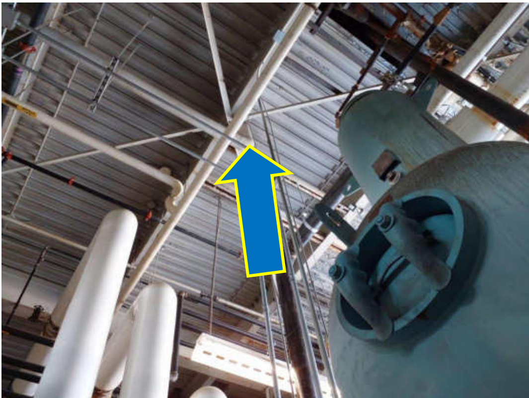
S0010 (Confirmed Asbestos), Piping, Parging Cement, Boiler Room (Location #: 1)
