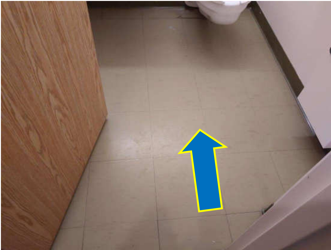
V0071 (Confirmed Asbestos), Green with black striations, Floor, Vinyl Floor Tile, Office (Location #: 292)
