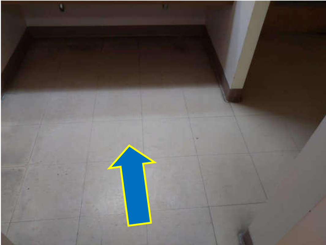
V0023 (Confirmed Asbestos), Floor, Vinyl Floor Tile and Mastic, Women's Washroom (Location #: 194)
