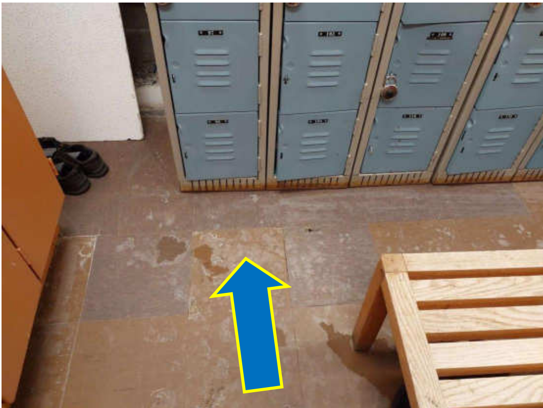
S0027 (Confirmed Asbestos), Floor, Vinyl Floor Tile and Mastic, Woman's Locker Room (Location #: 58) 10 sf abated as of 2025
