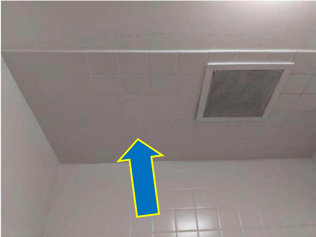
V9500 (Presumed Asbestos), Ceiling, Mortar, Storage (Location #: 125)
