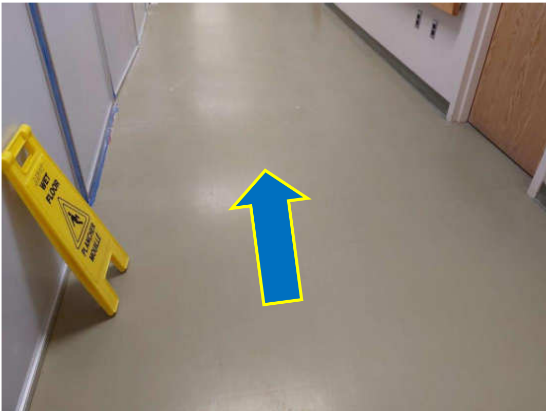
S0055 (Confirmed Asbestos), Floor, Vinyl Floor Tile and Mastic, Corridor (Location #: 184)
